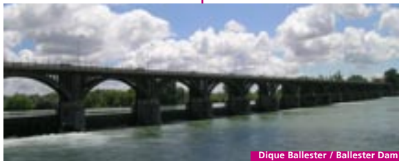
Dique Ballester / Ballester Dam
