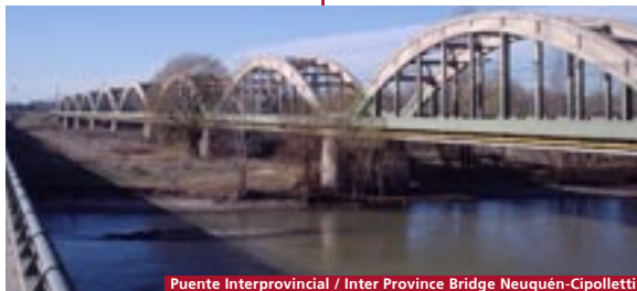
Puente Interprovincial / Inter Province Bridge Neuquén-Cipolletti
