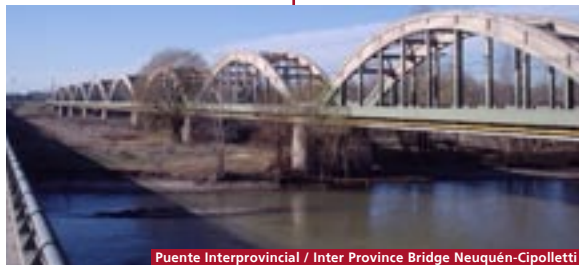
Puente Interprovincial / Inter Province Bridge Neuquén-Cipolletti
